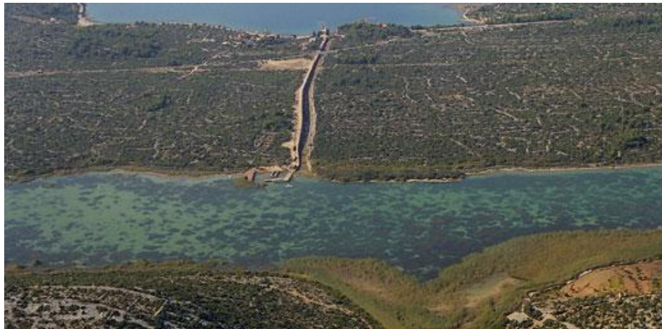
Figure 1.3 Aerial view of the Prosika canal. Abundant macrophyte vegetation near the shoreline can be noticed, confirming the vegetation-dominated clear state of the lake. NPVJ photoarchive.
